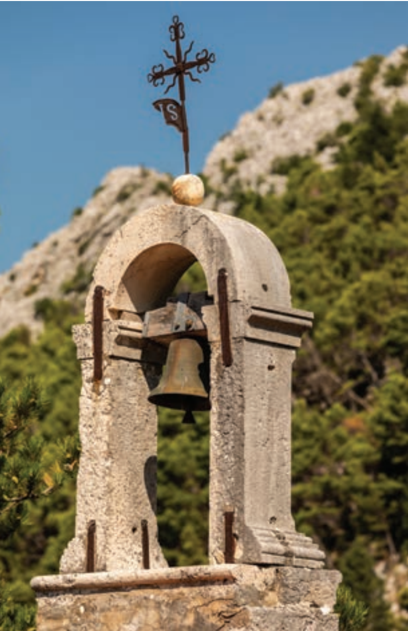
the bell-gable with one bell
